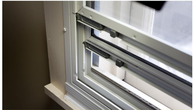
Tracked interior window panels are just like exterior storms, but permanently installed on the inside of the window. With integral screens, they adjust for ventilation. Made of glass, they are durable, clean easily, and are available with low-e coatings.
